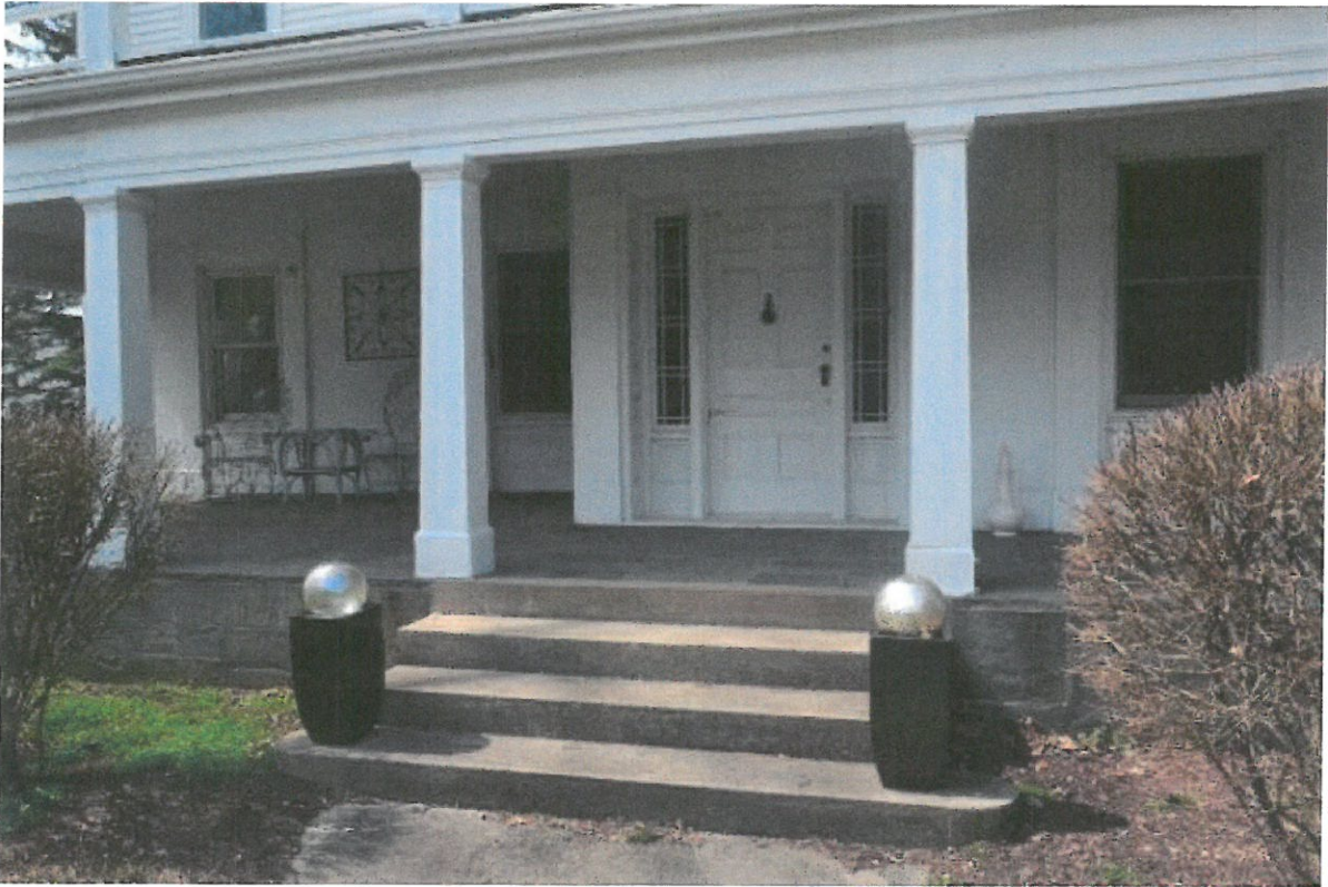
View of the front porch and entrance
