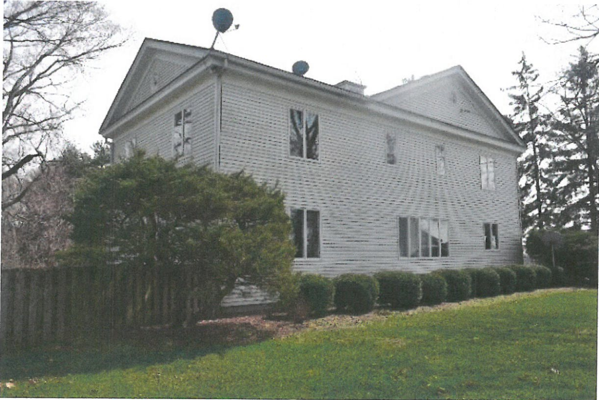
View looking Southeast to the West elevation
