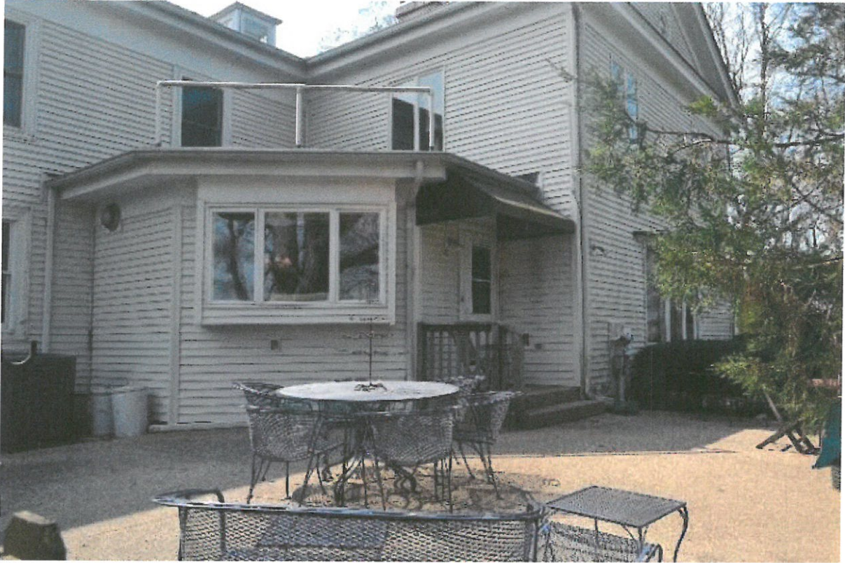
View of the patio and North elevation
