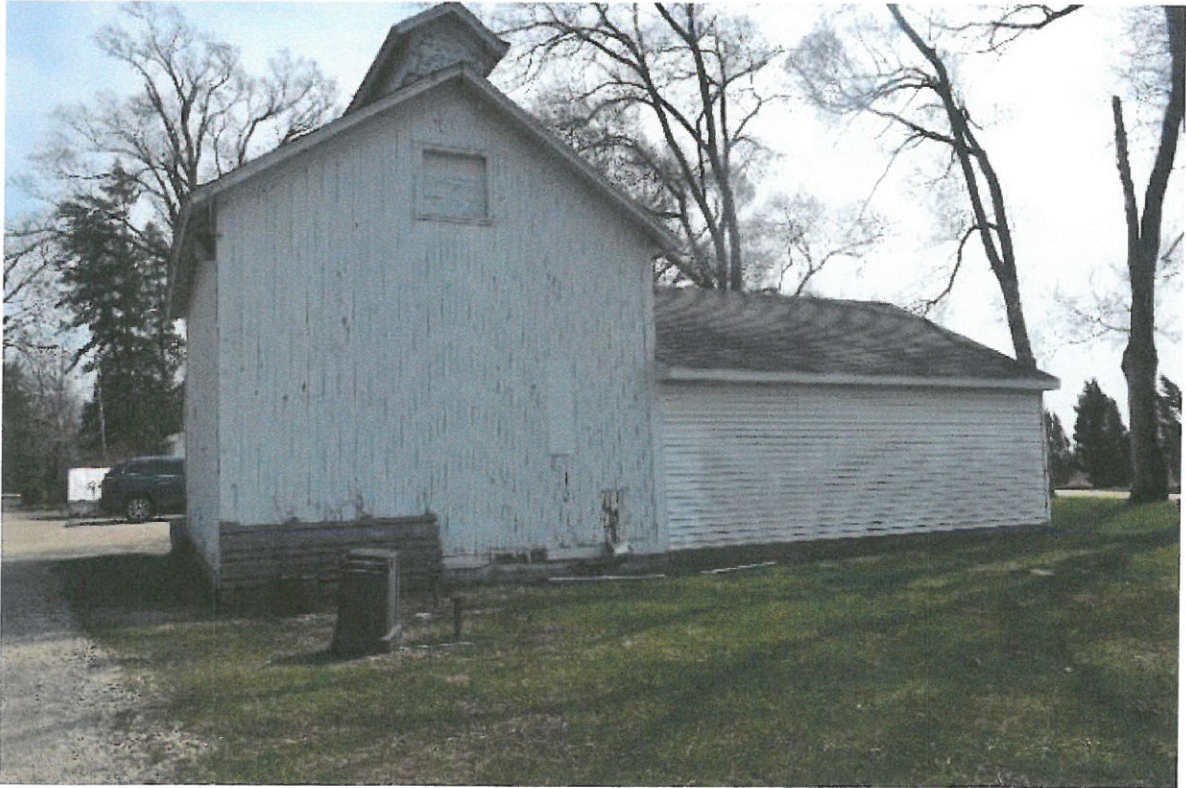
View of the storage barn
