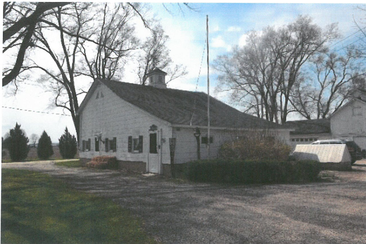
View of the apartment
