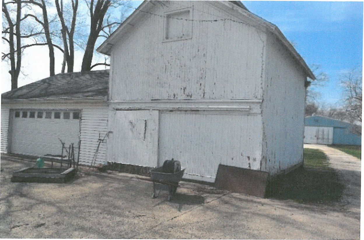
View of the storage barn
