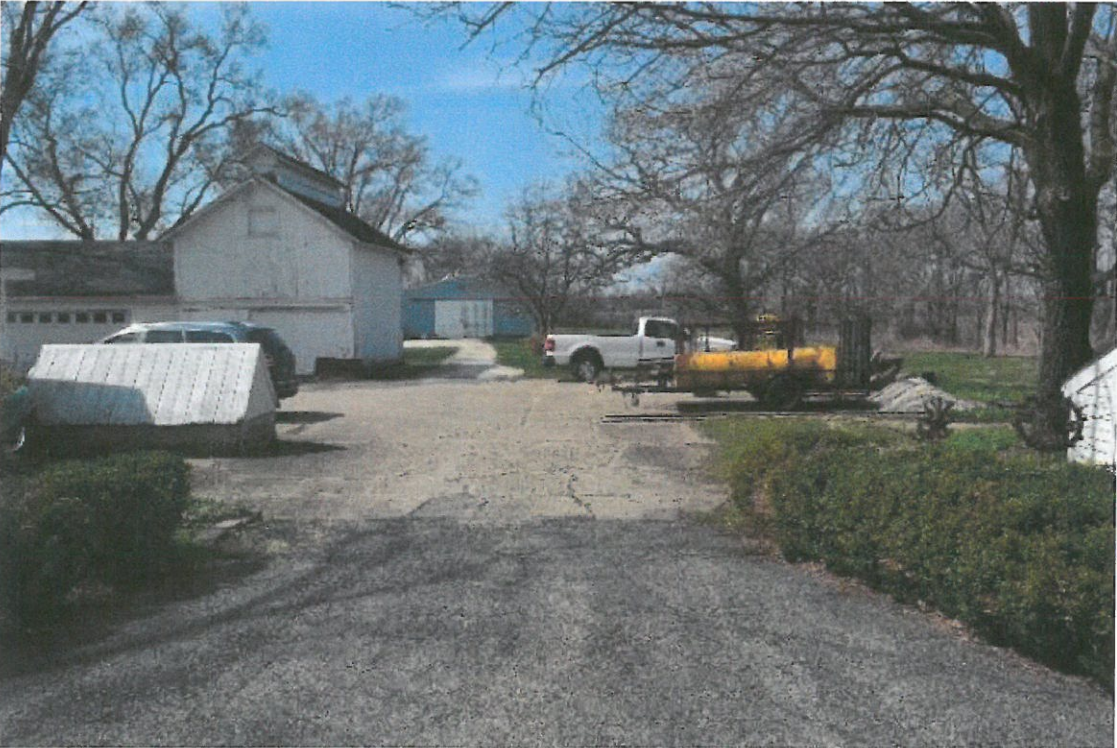
General view of the outbuildings
